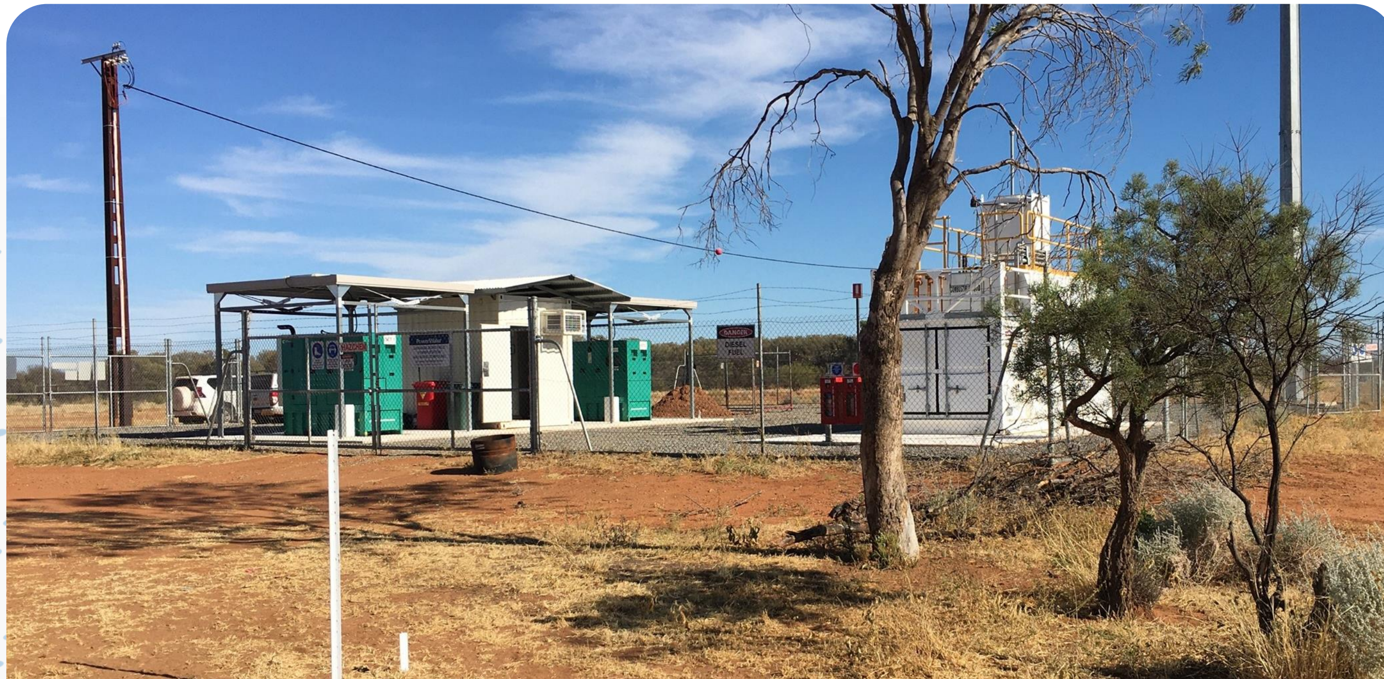
Photo of the existing water treatment site at Laramba
